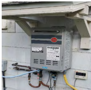
▲ A gas-fired flash water heater affixed to the building's exterior siding, making it part of the building and therefore covered.
