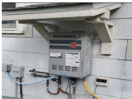
Figure 63: Wall-mounted Tankless Water Heater
