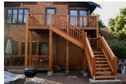
Figure 38: Deck with Single Set of Stairs
