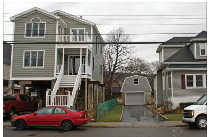
Figure 1: The house on the left is in the final stages of being elevated, which will result in reduced flood risk and lower flood insurance rates compared to the house on the right (Highlands, NJ)
